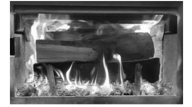
Close the primary air control by small increments (ex: 1/16 of an inch) until reaching the midpoint of air control position, between 4 and 15 minutes after the loading period. Before closing further, make sure the flame intensity is increasing or stable. Turn ON the blower at maximum speed.
