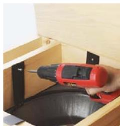
4. Once the support is secure, you can begin to assemble the chimney by lowering the first section into the support. Make sure that the male coupler is pointing upwards, as indicated by the arrow on the chimney label.
